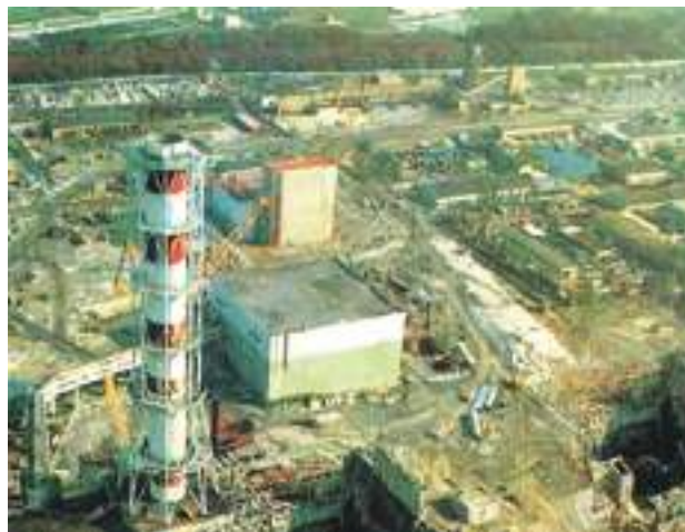
Chernobyl nuclear power plant after the explosion
